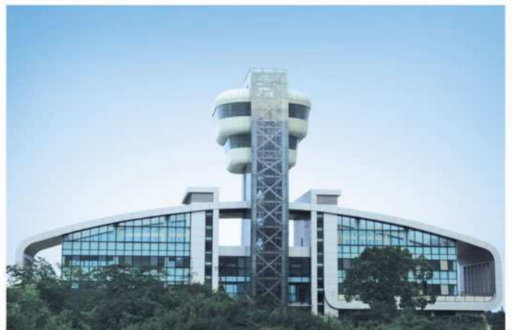
Jiangsu Shuofang International Airport
